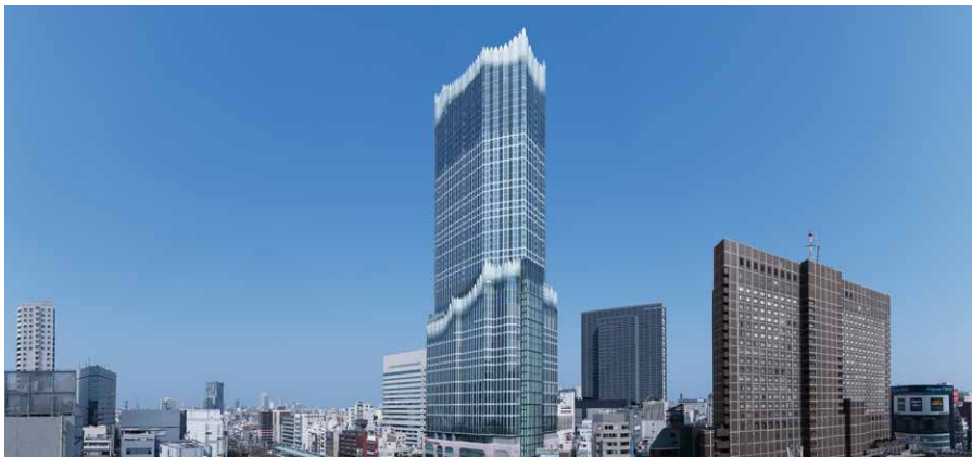
©TOKYU KABUKICHO TOWER
